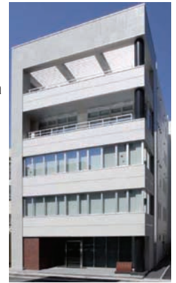
Keisoku Kaikan Building
