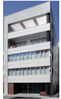
Keisoku Kaikan Building
