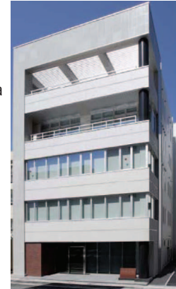
Keisoku Kaikan Building
